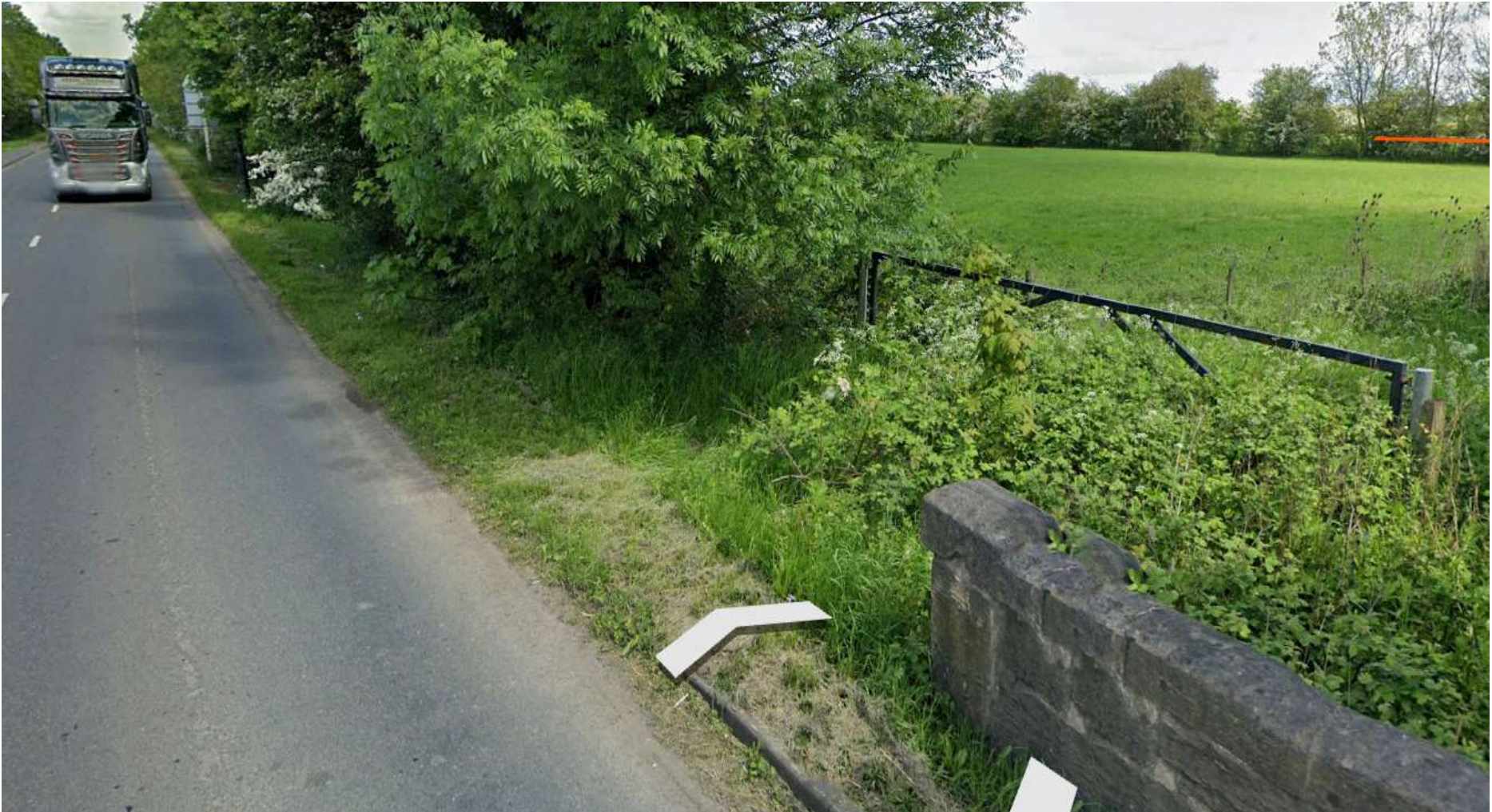
D - Image showing view of entrance to car park A from the South
